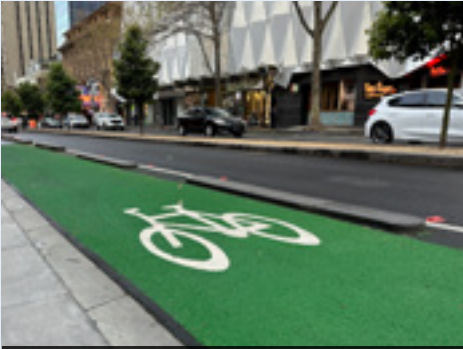
We've installed wider footpaths and safer bike lanes in the Exhibition Street theatre precinct
